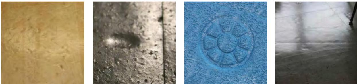
It is seldom that hard-surface flooring indentations are the result of flooring material failure. The source of indentations can typically be traced back to installation error, installation system failure, point loads exceeding the flooring system limits or an extreme environment that compromises the flooring. Most important, the flooring manufacturer is usually NOT the culprit when delegating blame and looking for someone to pay for corrective measures.
