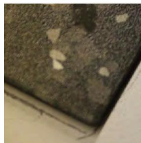
*Photo 8: With 3-1/2" subfloor deviation, tile alignment shifts drastically.*
