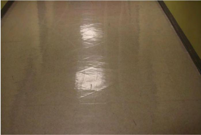
*Pattern of existing floor shows through the new floor even though the underlying material should have been removed according to flooring manufacturer instructions.*
