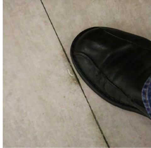
*Excessive moisture coming up from the slab beneath the floor due to vapor emissions that exceed allowable level.*
