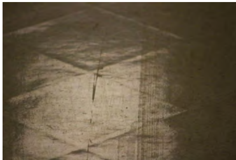
When laying new resilient sheet over existing vct floor tiles, results are not always good due to existing conditions.
